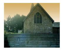
This 13th Century listed building was in danger of subsiding into the River Teme as the bank was eroded below the church. Construction of a five metre high reinforced concrete retaining wall was required to underpin the existing structure at river level. Anchored by stainless steel ties to concrete blocks set 20m back from the wall face, the work necessitated the strengthening of the existing concrete apron.
